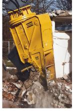
primary demolition of light- to medium-reinforced concrete structures, secondary reduction and material separation. The unit's replaceable blades effectively cut rebar as the tool penetrates through concrete. The blades are reversible to provide longer service life.
